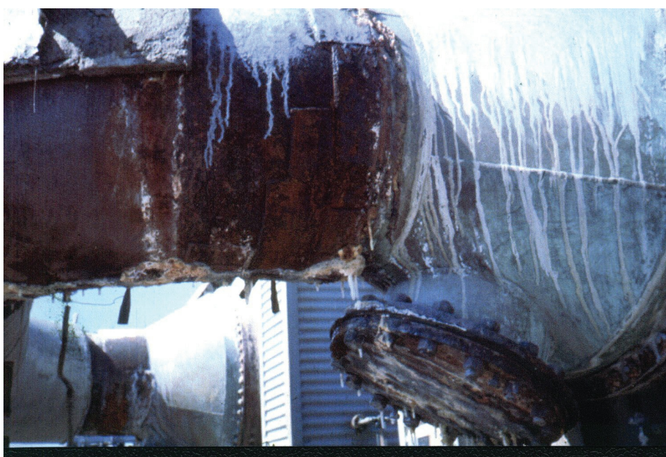
FIGURE 1.3: Water box and feed water pipe for a heat exchanger from a multi-stage flash desalination plant.
