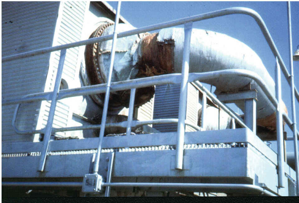
FIGURE 1.1: Piping and inlet water box for a multi-stage flash desalination plant.
